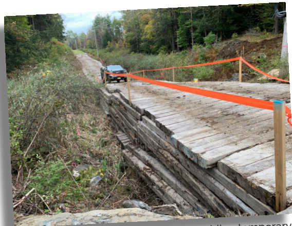
Layered wetland matting providing temporary wetland crossing
