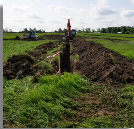
Tile drain removal for wetland restoration, Ducks Unlimited
