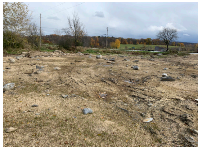
Post restoration-fill removed, rough finish incorporating boulders
